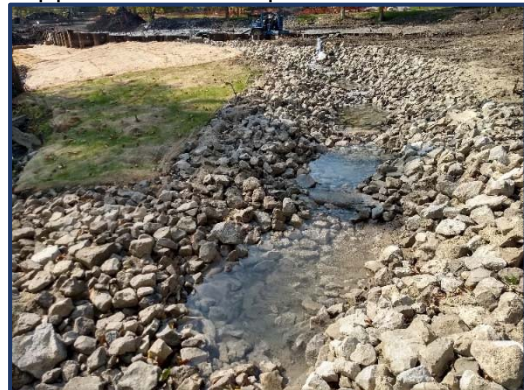
October 9, 2020 Step pool construction complete
